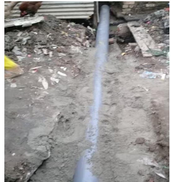
Pipe laying in the lane
