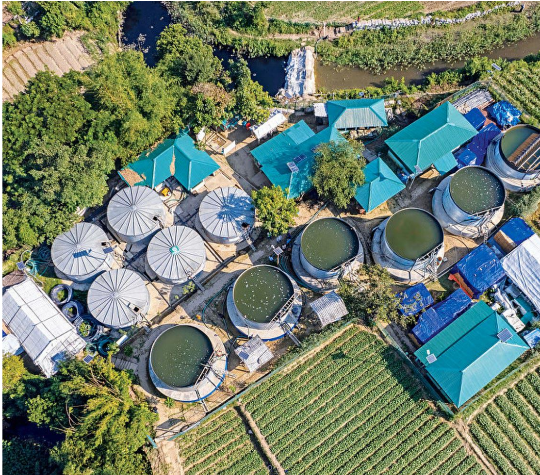
Surface Water Treatment Works (SWAT)
